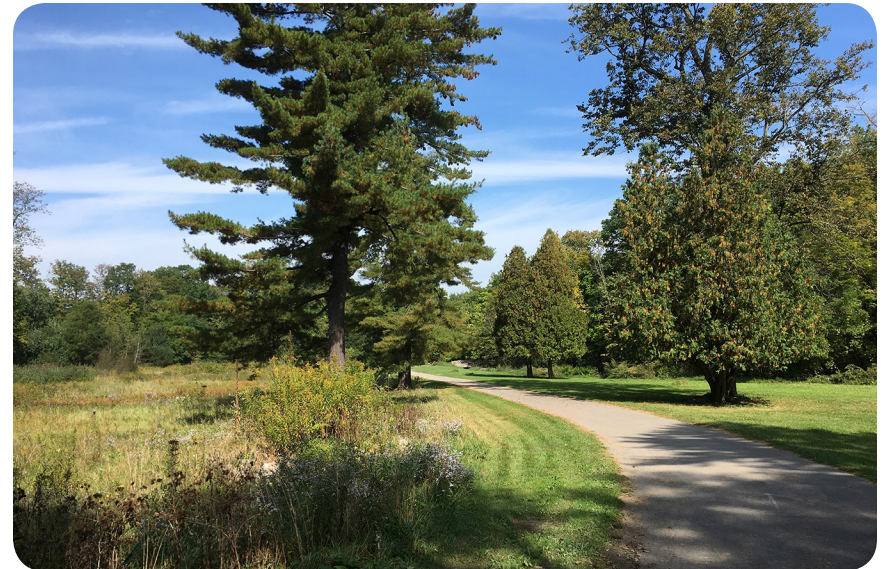
Asphalt paved roadway/pathway, F. T. Proctor Park
