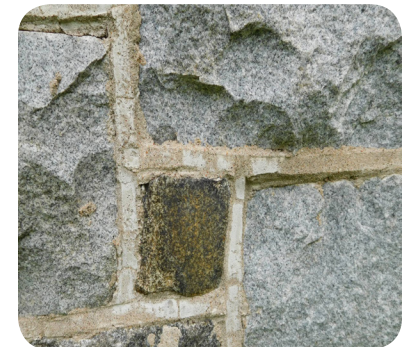
Mortar joint tooling
