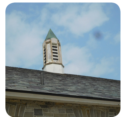
Roof vent and slate roofing
