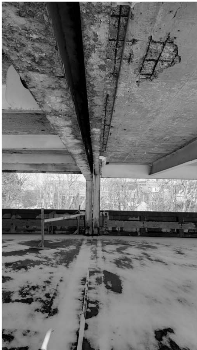
Expansion joint, spalled south wing concrete above
