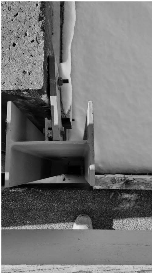
Separation gap of north wing southwest corner column
