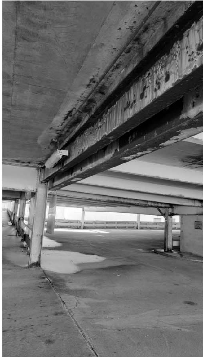
Second floor joint and corroded existing beams above
