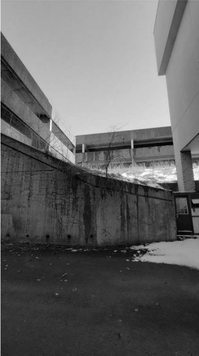
Cantilever retaining extension wall, west end of tunnel South end of north wing (Left) at corner intersection with south wing of garages (Center) Hospital (Near right)
