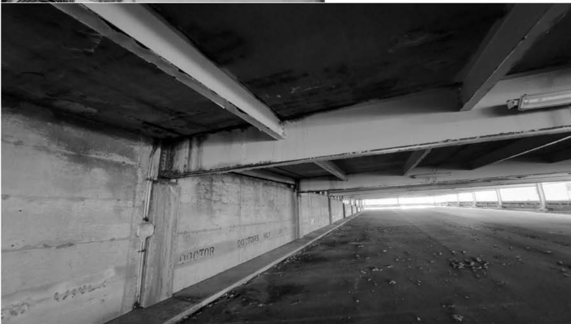
Mid-width South Wing Retaining Wall running east to west and existing corroded steel beam.
