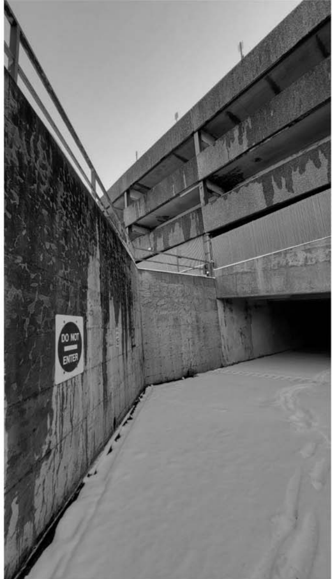
Cantilever retaining extension wall, east end of tunnel
