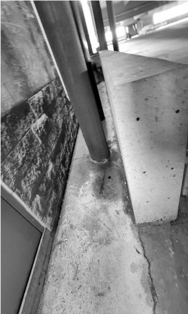
Northwest hospital access door & crack at joint (Both Photos)
