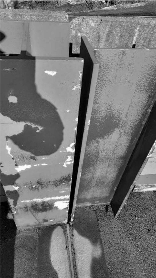
Double Column separation at roof east edge
