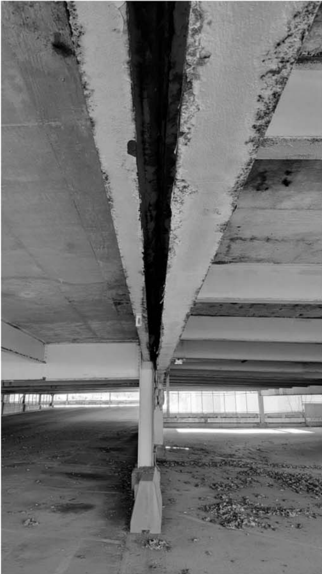
Ground level slab joint and double beam above
