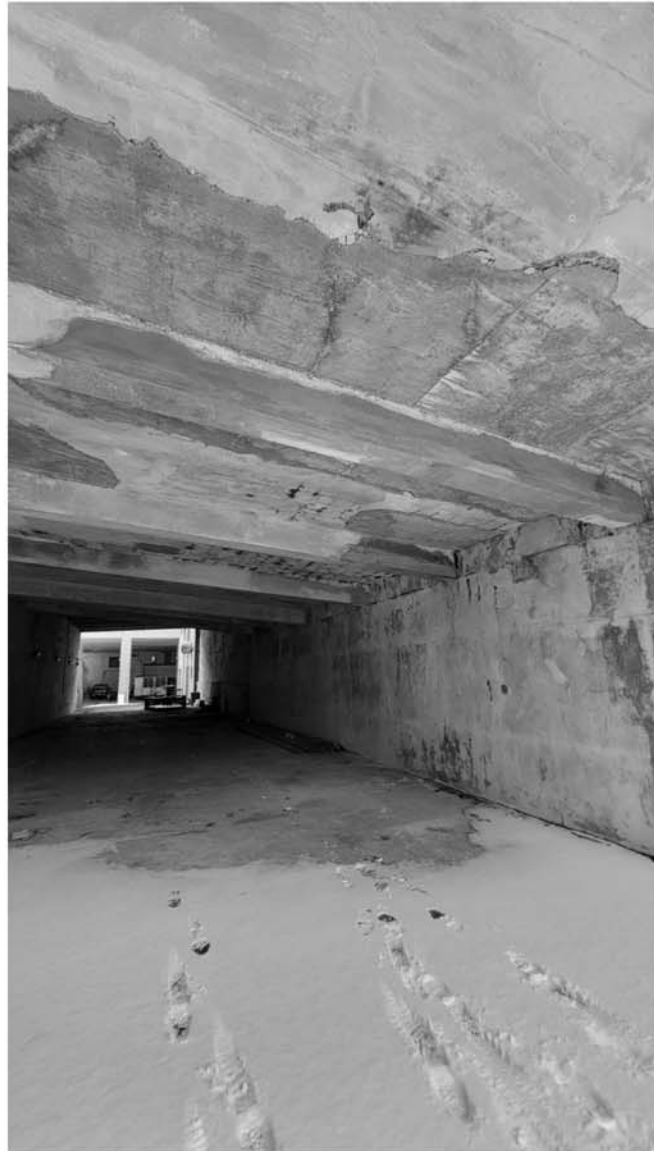
Tunnel East beams North wing corrosion & patches
