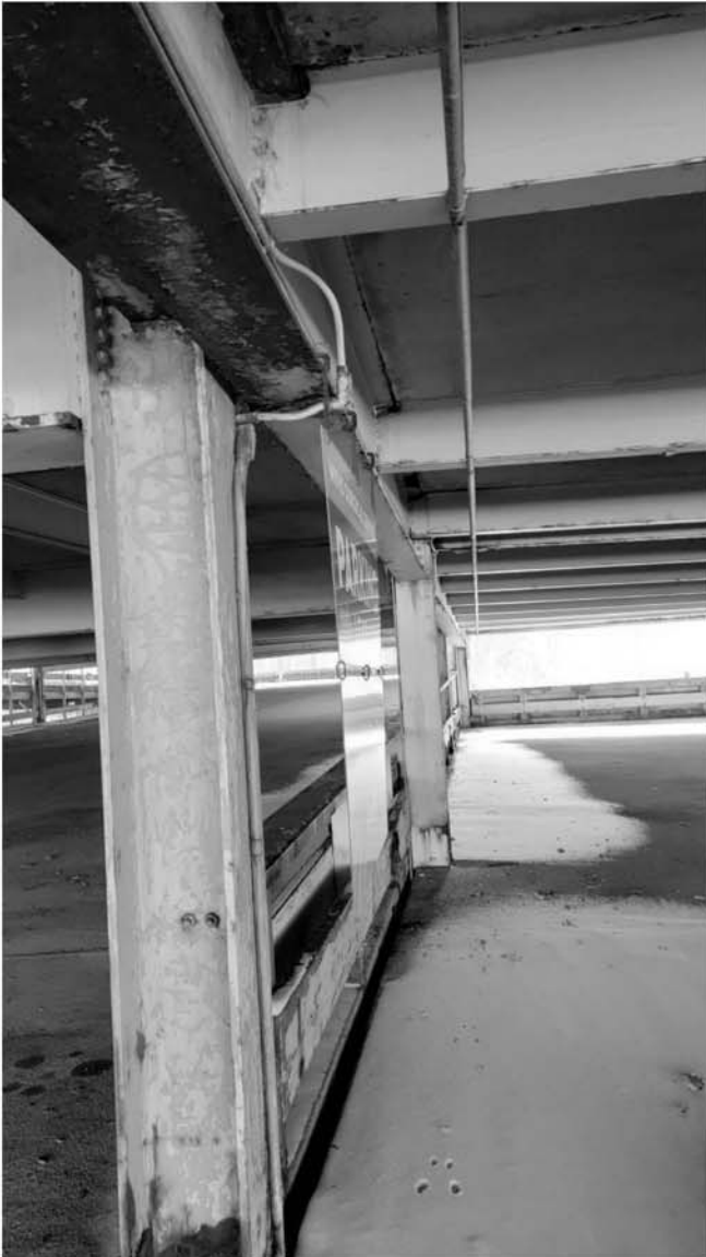
Second floor joint and staggered existing column grid
