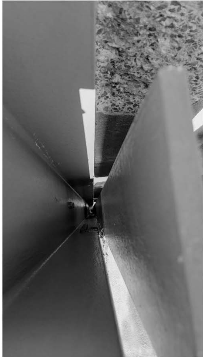
Full Height Separation at Double column
