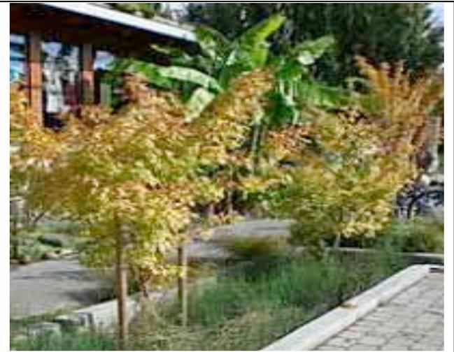
Also known as infiltration swales, biofilters, grassed swales, or in-line bioretention, bioswales are vegetated open channels specifically designed to attenuate and treat stormwater runoff for a defined water volume. Bioswales intentionally promote slowing, cleansing and infiltration along the way, thereby reducing runoff volumes into the Utica stormwater systems.
