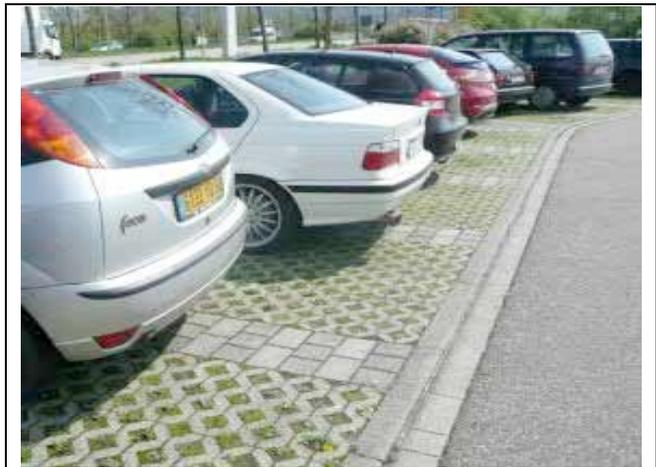
Permeable pavement can be used instead of standard asphalt and concrete for surfacing sidewalks, driveways, parking areas, and many types of road surfaces.
